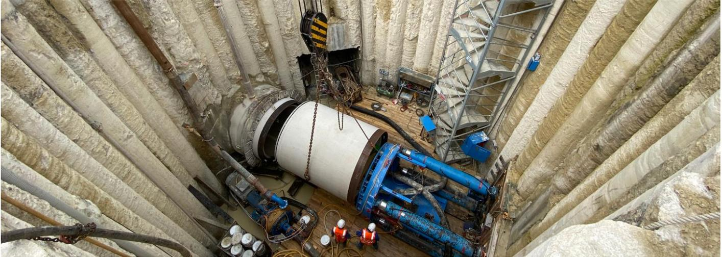
In the densely populated city of Gagny, just outside Paris, a large water collector was built by the use of microtunneling. This basin will serve as a rain collector, avoiding floodings in the event of heavy and long rain periods.
